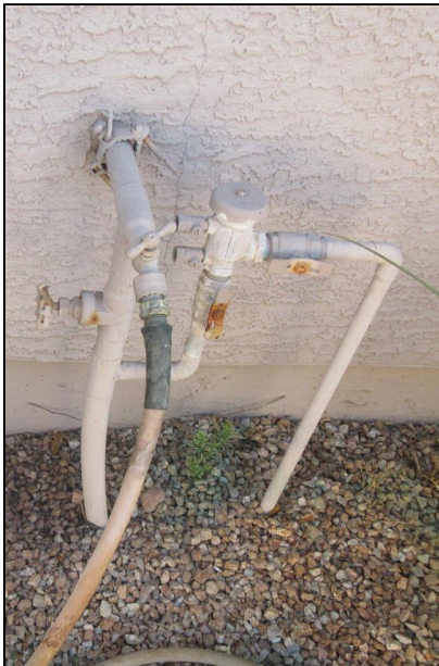
5.1 Item 1(Picture) Water main shut-off southeast front corner of home
