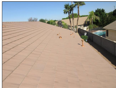
4.0 Item 2(Picture) North facing roof covering
