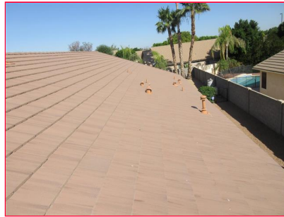
4.0 Item 2(Picture) North facing roof covering
