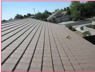
4.0 Item 1(Picture) South facing roof covering
