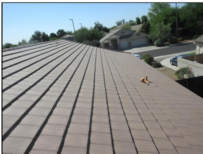
4.0 Item 1(Picture) South facing roof covering
